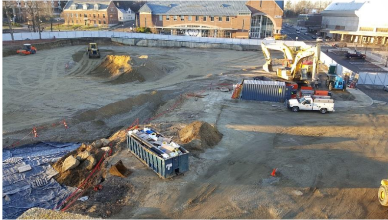
Site preparation for upcoming building project
