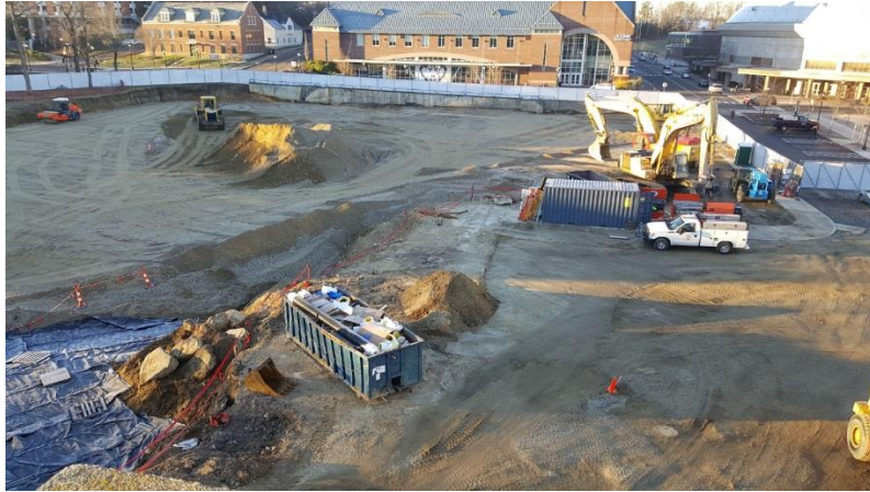
Site preparation for upcoming building project
