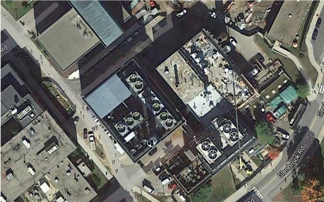
Central Utility Plant and project cooling towers at right
