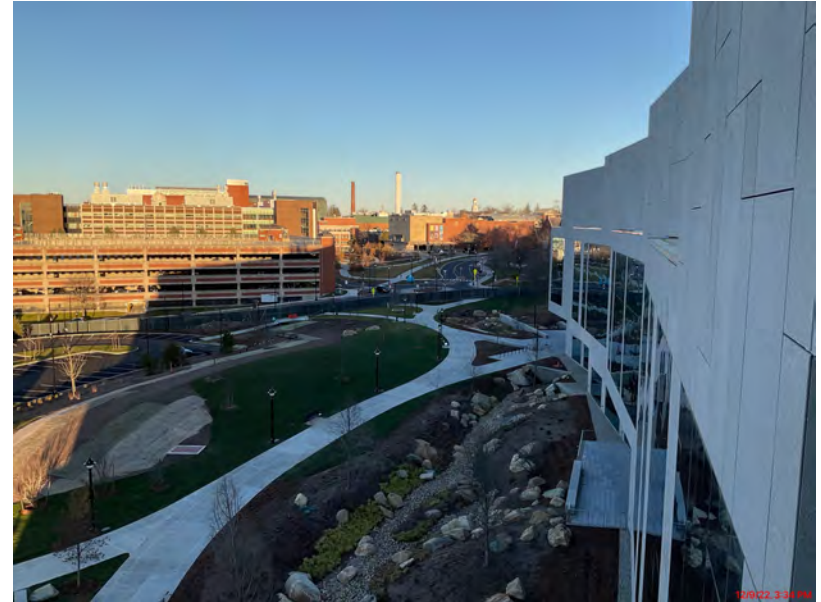
North Elevation Looking East
