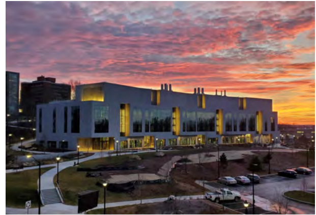
North Elevation Looking South
