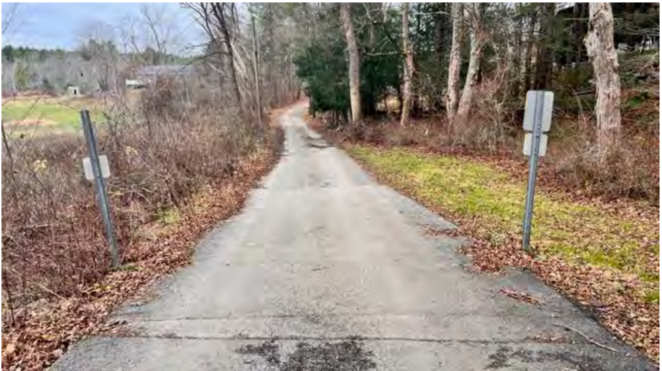
Pumping Station Road Looking East Towards Gurleyville Road
