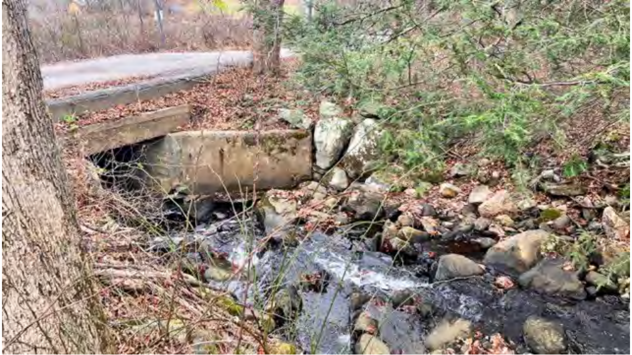
Looking North into Existing Culvert
