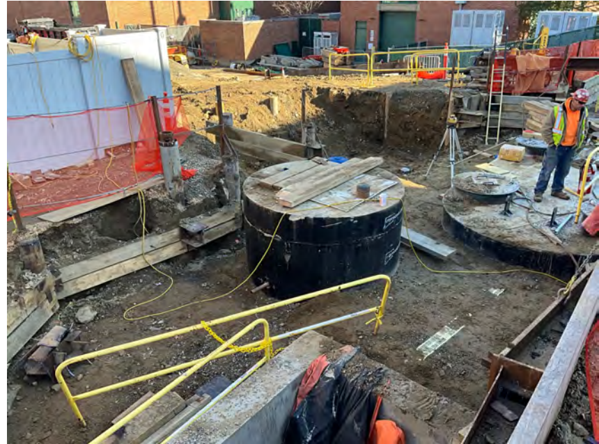
B4 Steam Vault Installation
