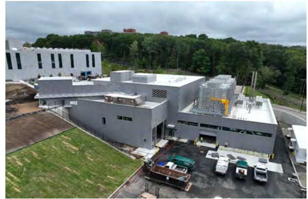
SUP View Looking South
