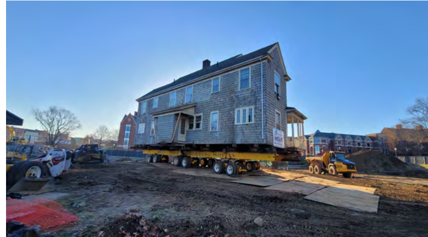
4 Gilbert Road House Relocation
