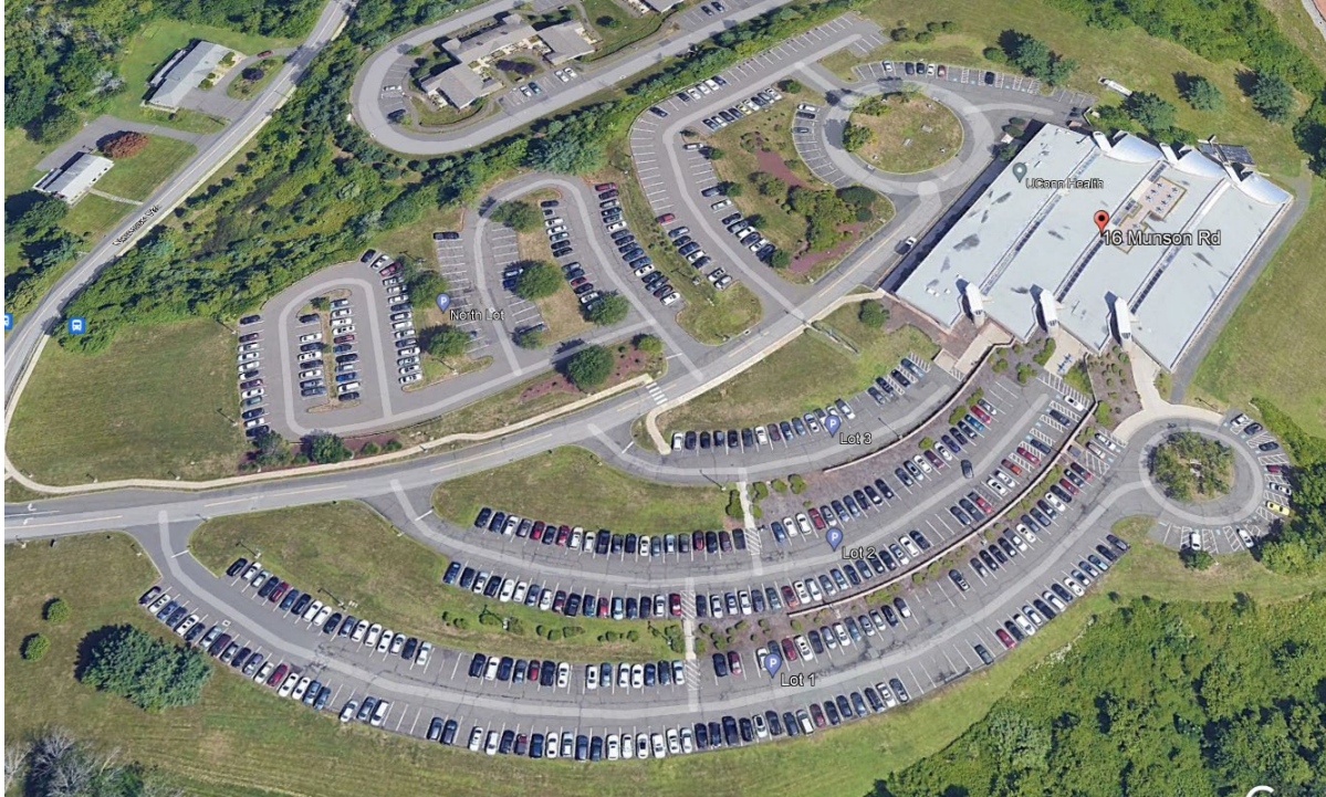
16 MUNSON ROAD PARKING LOTS
