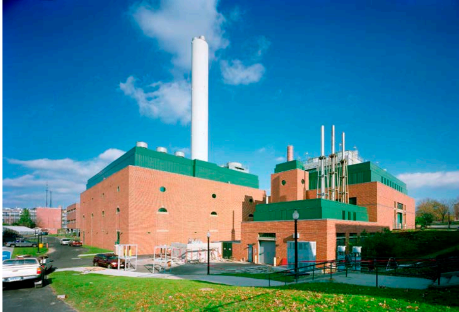
Existing Central Utility Plant
