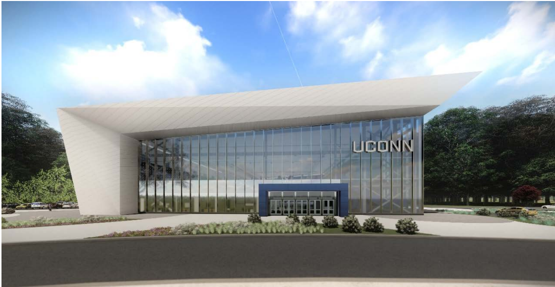
Northwest Elevation along Jim Calhoun Way
