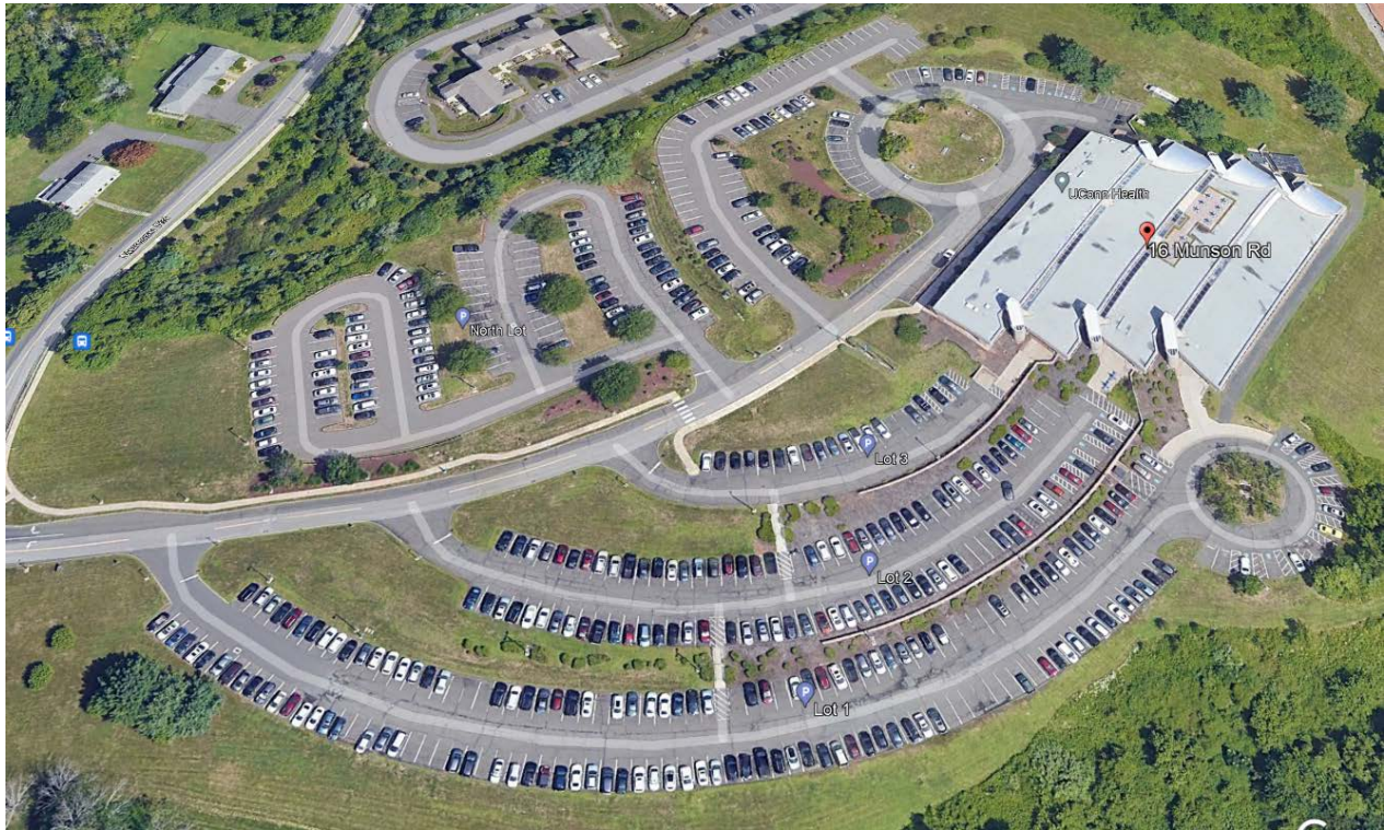
16 MUNSON ROAD PARKING LOTS
