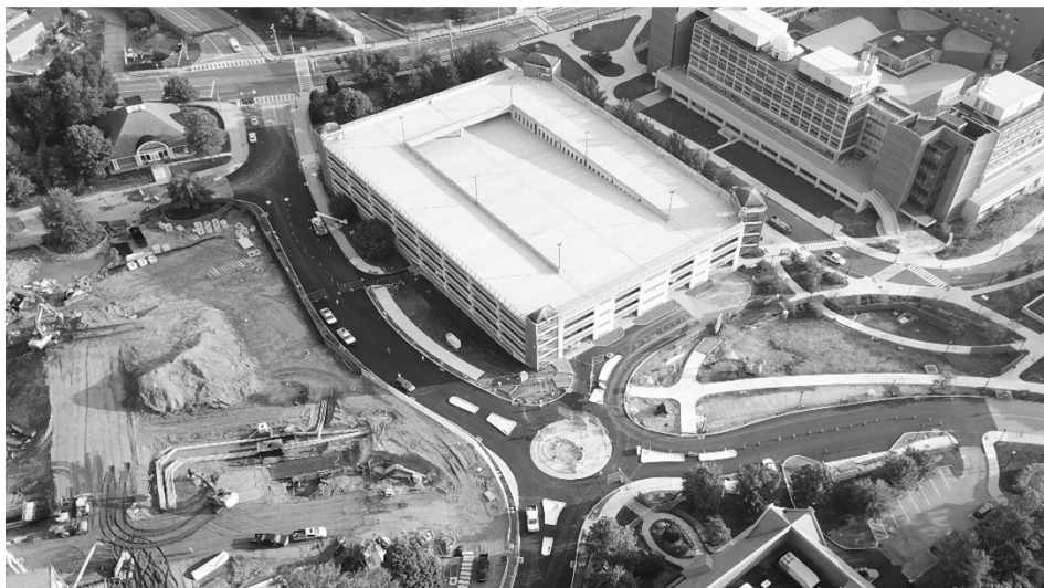
Supplemental Utility Plant
