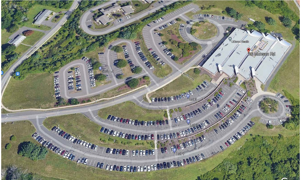
16 MUNSON ROAD PARKING LOTS
