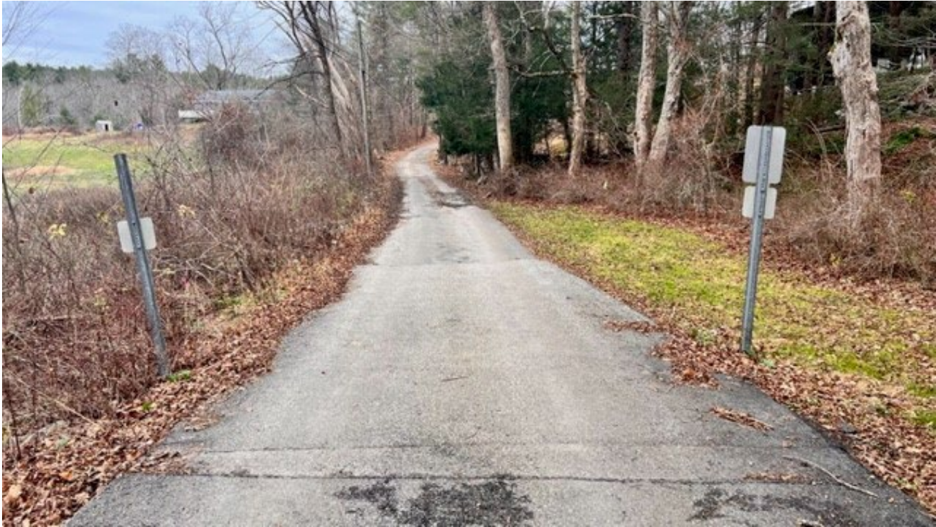
Pumping Station Road Looking East Towards Gurleyville Road
