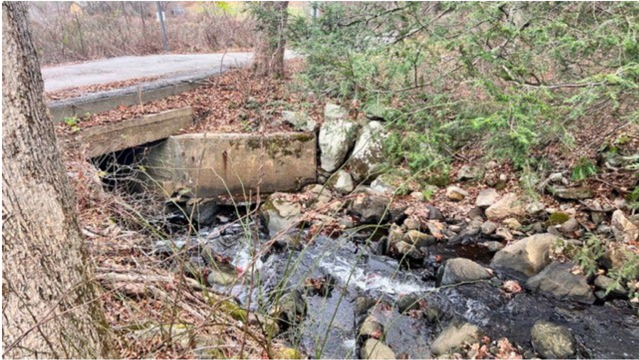
Looking North into Existing Culvert
